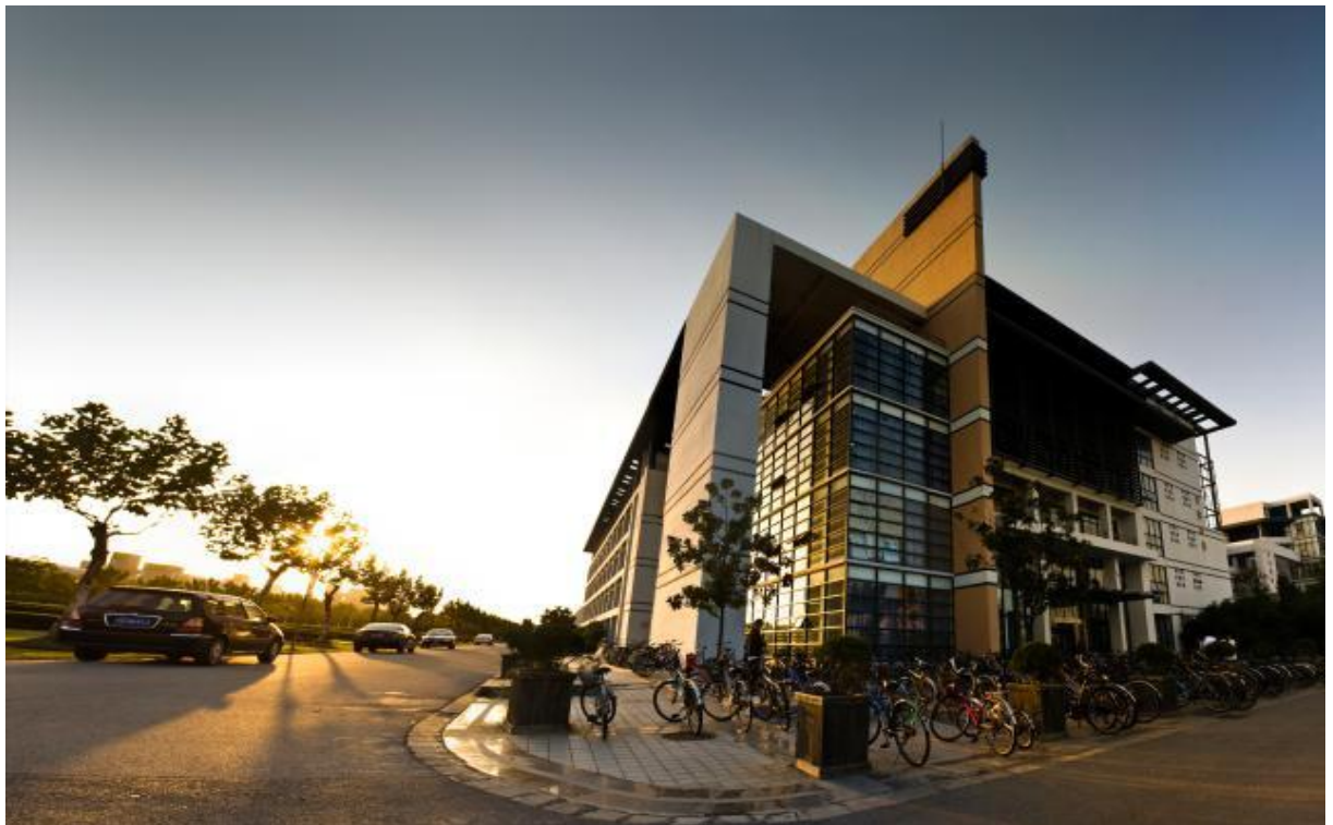
信息学院大楼 Building of College of Information Science and Technology
